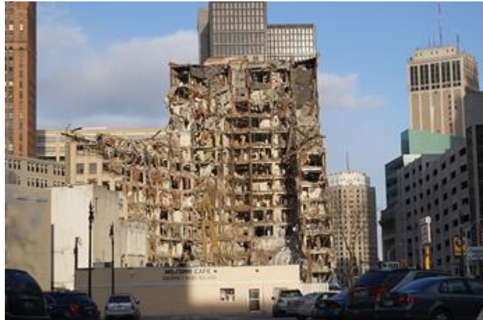
Figure 1 Lafayette building, former seat of Michigan Supreme Court (commons.wikimedia.org / gemeinfrei)
